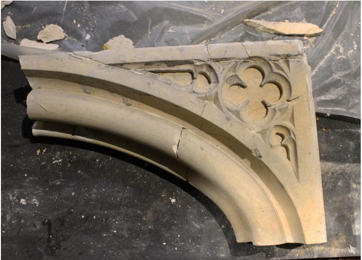
Top: arch section being repaired. Bottom: the iron elements removed from the monument
